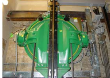
Gearless Hoist Motor
