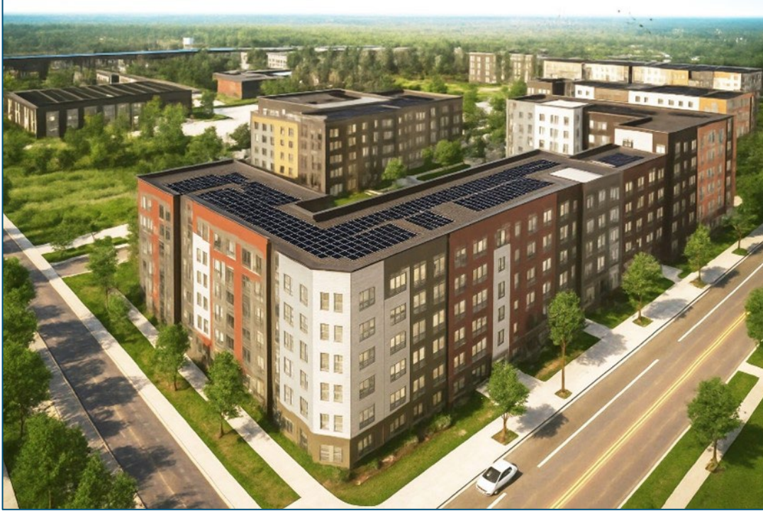
The Heights Geothermal District Energy System
